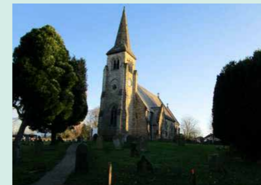
Photo 8: View of St Mary's Church
