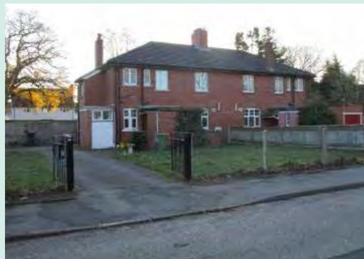
Photo 16: Housing on south side of Alexandra Road
