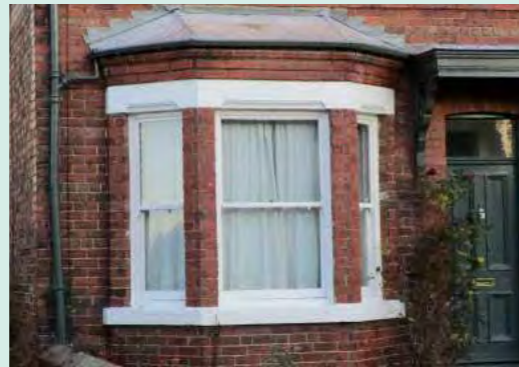
Photo 41: Example of a single colour smooth red brick
