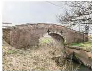
Strensall New Bridge - Haxby Moor Road
