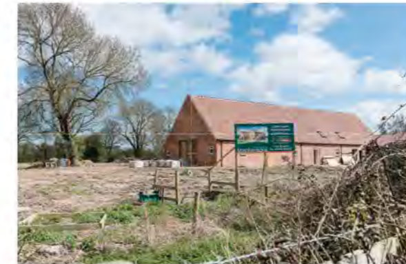
Towthorpe: conversion of agricultural buildings
