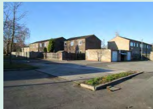
Photo 19: Housing to the north of Howard Road
